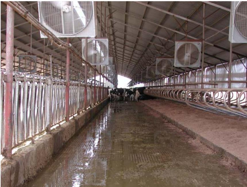
First, if you need to add or replace fans before summer heat strikes, include energy efficiency as a criteria when purchasing new ones. The Bioenvironmental and Structural Systems Laboratory (BESS), an independent laboratory at the University of Illinois, conducts performance tests of equipment. In their tests, they found considerable variation in the amount of air delivered and the energy efficiency for both 36" and 48" fans (Table 1).
